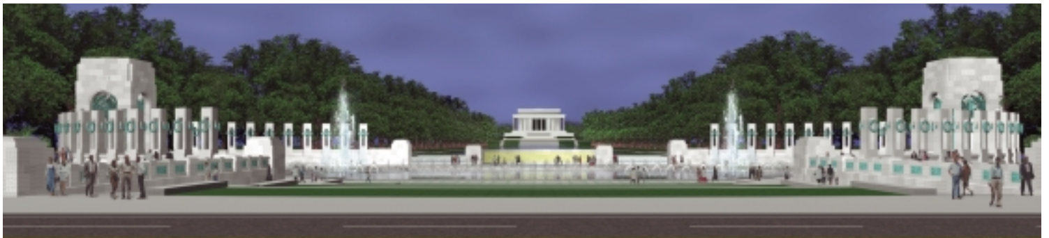
View of the memorial from 17th Street showing open vista to Lincoln Memorial
